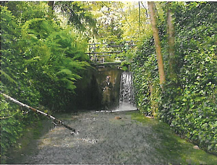
Figure 12: Diversion dam on North Fork Tuttle Creek.
