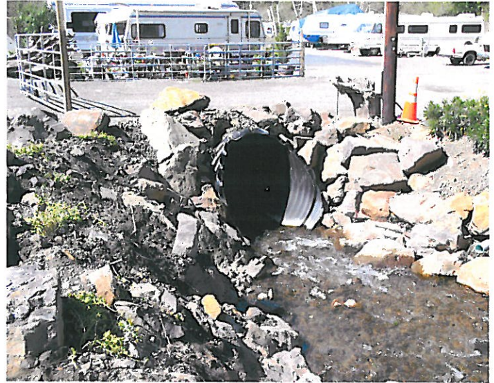
Figure 10: Upper R.V. park culvert
