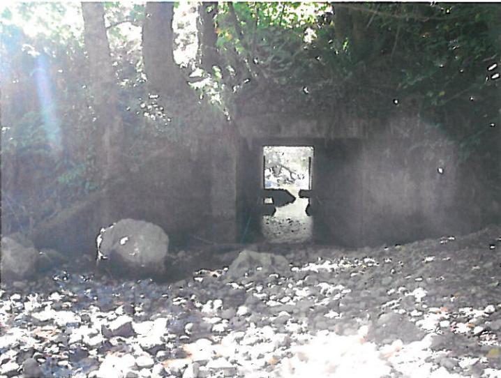
Figure 16: Joe Hall Creek Culvert Inlet
