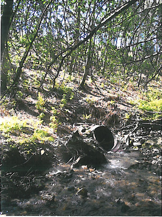
Figure 3: U.S. 101 Culvert Inlet
