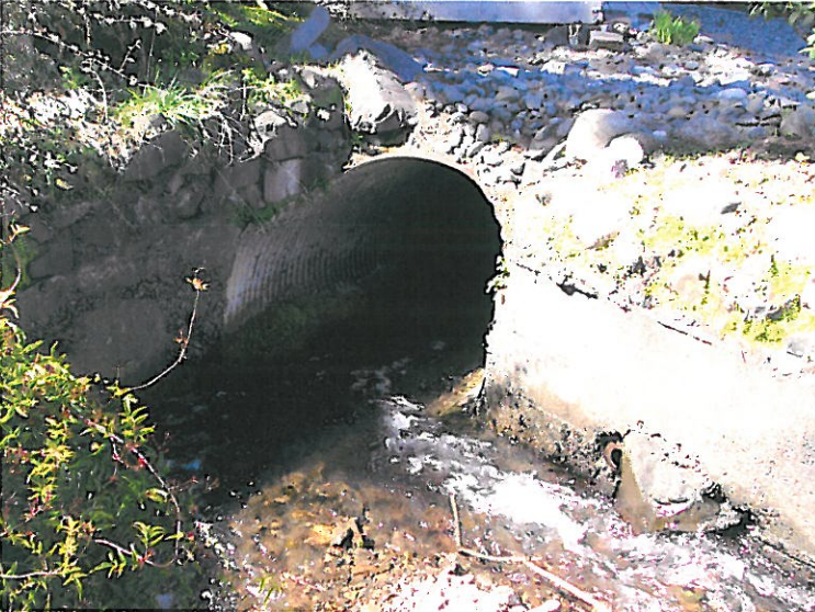
Figure 8: Inlet of lower R.V. Park culvert
