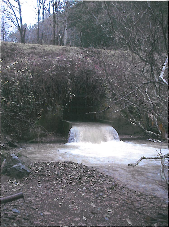
Figure 17: Joe Hall Creek Outlet: Winter Flow
